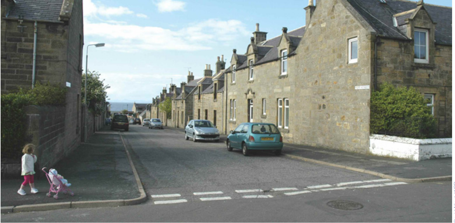
Quadrant kerbstones used instead of large radii at junctions reduce the dominance of the carriageway and respond to pedestrian desire lines – this is reinforced by the placement and form of the adjacent buildings
